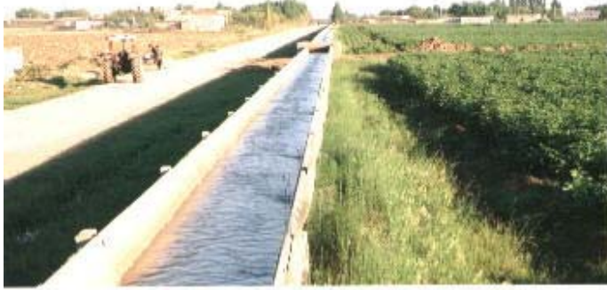
Water Canals in Southeastern Turkey
